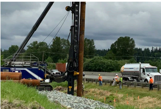
Subsurface Construction, an MBE firm, played a key role in ensuring the new bridge has a solid foundation. Here they are installing some of the piles that will support the bridge.
