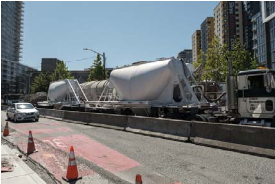
Battery Street Tunnel decommissioning: Low density cellular concrete mixing plant staged along Borealis Avenue, just south of Denny Way
