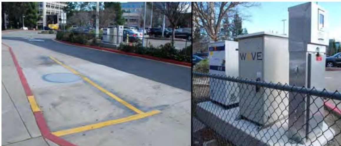
Figure 26: Inductive Charging Infrastructure (Courtesy: WAVE)
