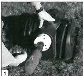
Drill endcap on side or top.
