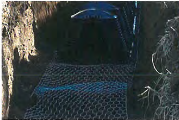
Figure 1a: Roll out chicken wire
