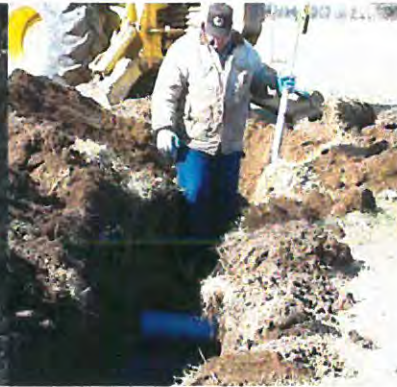
Figure 1b: Install chambers over the wire base
