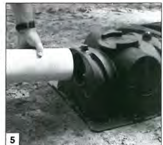
Insert inlet pipe.
