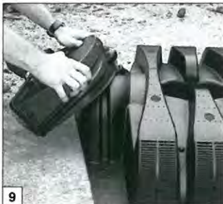
Place end cap outlet end.
