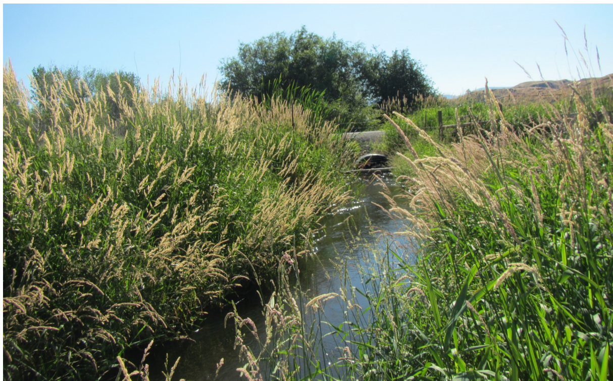
Photo 3. Representative channel condition, and Conconully Highway culvert.
